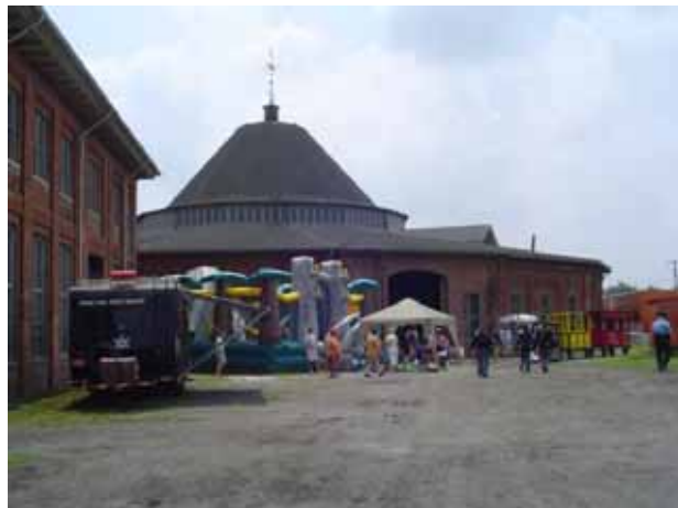
Significant improvements were made to the roundhouse and adjacent structures. Photo by R. Rodriguez
