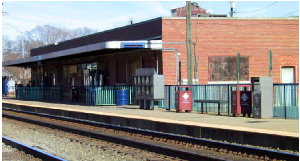
Quantico Train Station is currently undergoing renovation.
